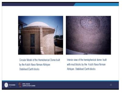
Also, some of the circular models which is a hemispherical dome. This is completely done with the bricks, you know with the mud blocks.
