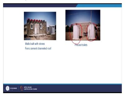
And the Ferro-Cement Channels which I have showed you just now how they are fabricated and some of the houses were also constructed on that and as well as some toilets, you can see that these are the precast toilets, toilet units so these are some of the interventions, some ideas because this whole disaster becomes the follow-up of this becomes a kind of place a laboratory of different ideas and experiments.
